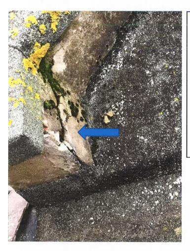
Further photos of the west facing bay. The render on the wallhead is cracked and will be letting in water.
