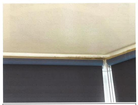
The photo above shows the water ingress to the smaller west facing bay window. The photos below show some of the causes; the felt is coming away from the coping stones and there joints are coming apart as the key demonstrates. **The owners have decided to leave this roof for now.**
