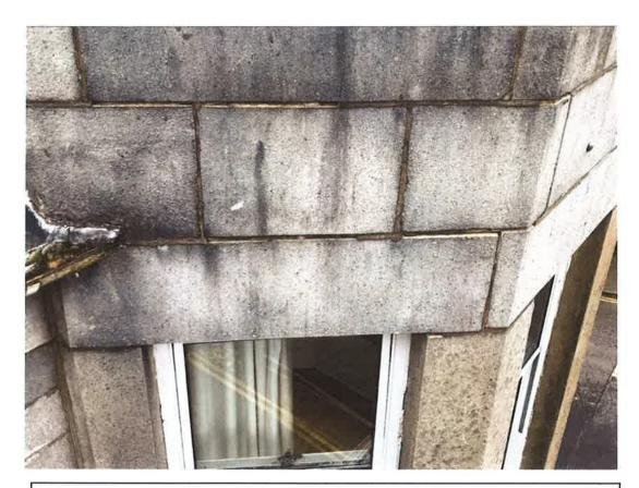
The top photo shows some of the failed pointing. The bottom left shows the left hand watergate which will need to be renewed with the flat roof.
